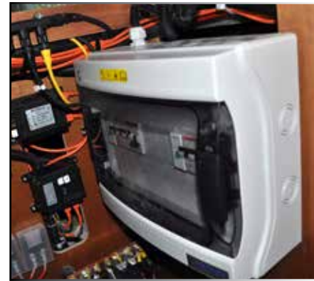
SET OF AUTOMATIC BREAKERS (110 V – 220 V)
