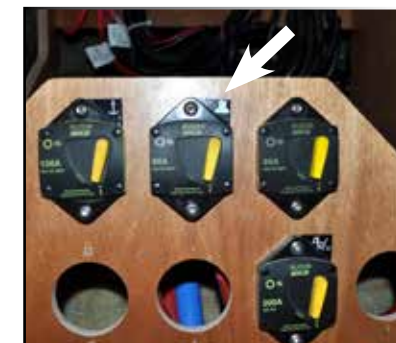
AUTOMATIC BREAKERS FOR THE ELECTRIC WINCHES
