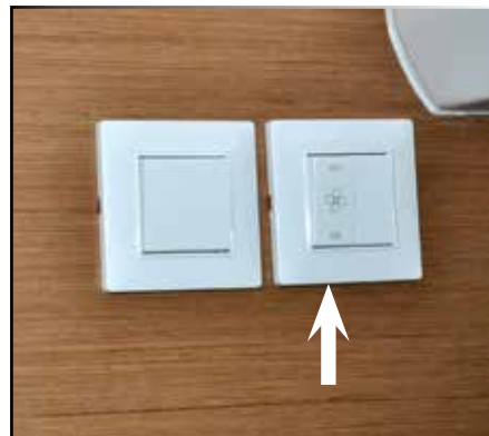
SWITCH FOR AIR VENTILATION OF THE AIR CONDITIONING SYSTEM (CABINS)
